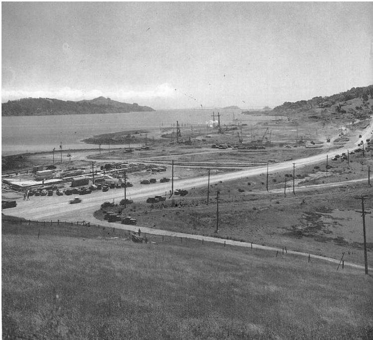
**Figure 67. Marinship site being filled and graded, spring 1942.**
