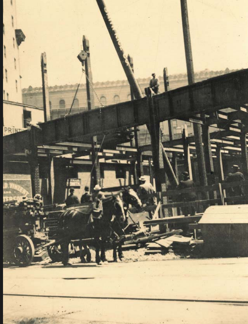
Steel frame being erected Image courtesy of the Mechanics' Institute
